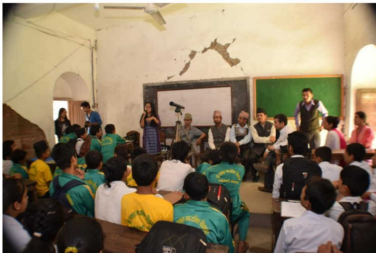
Photo 3: Benajil Rai asking questions to the students in side of Cracked building
